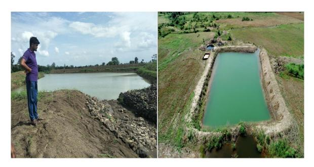
**Check dam & Stop Dam**– Efforts made to construct 8 Check dam & 1 Stop dam in 7 villages which will help to conserve water for dry season & lifesaving irrigation. (Conservation Estimate – 1, 14,300 Cum additional water Storage, irrigating 92 hectare Rabi crop additional for 66 farmers)
